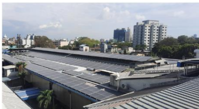
1.8 MW Solar system installation at Colombo site - to be connected
