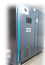
Installation of VSD compressor for PMD
