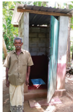
325 toilets built to improve sanitation
